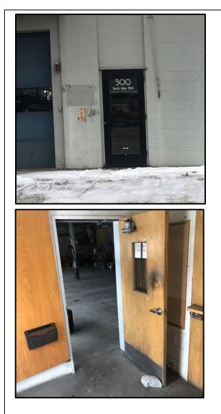
The main entrance door is too heavy and does not meet our accessibility requirements; therefore the door must remain open.
