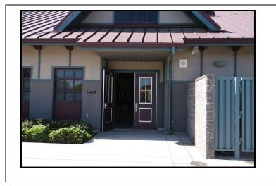
The entrance door(s) are too heavy and do not meet all the accessibility requirements; therefore the door(s) must remain open.
