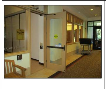
The entrance door to the Terra Cotta Room is too heavy and does not meet all the accessibility requirements; therefor the door must remain open.
