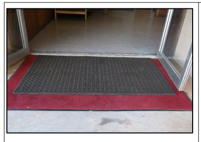
The threshold on the exterior side of the entrance is too high and does not meet accessibility requirements. Based on previous notes from this location, our threshold mats create a tripping hazard.
