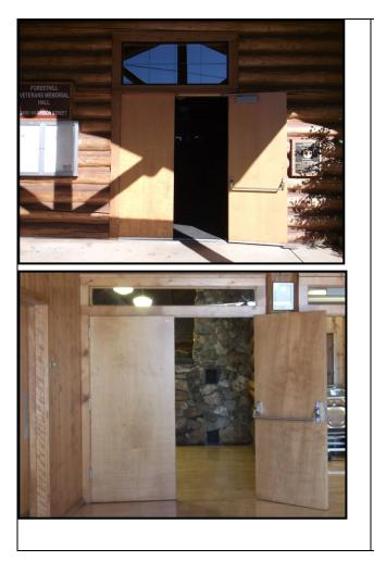
The main entrance doors and the interior doors are both too heavy and do not meet all the accessibility requirements; therefore the door(s) must remain open.
