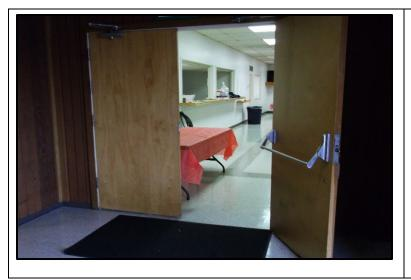
The interior door(s) to the community hall do not have accessible hardware and are too heavy and do not meet all of the accessibility requirements. The door(s) must remain open.
