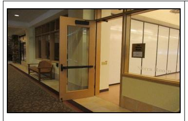
The door into the Sierra Room is too heavy and does not meet the accessibility requirements; therefore the door must remain open.
